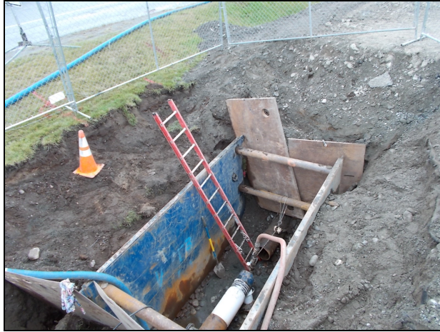
Figure 4. Typical liner access pit
