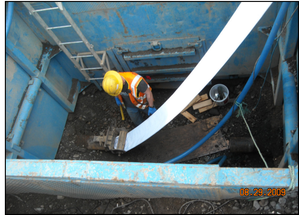
Figure 9. CIPP insertion into an AWWU cast iron main.
