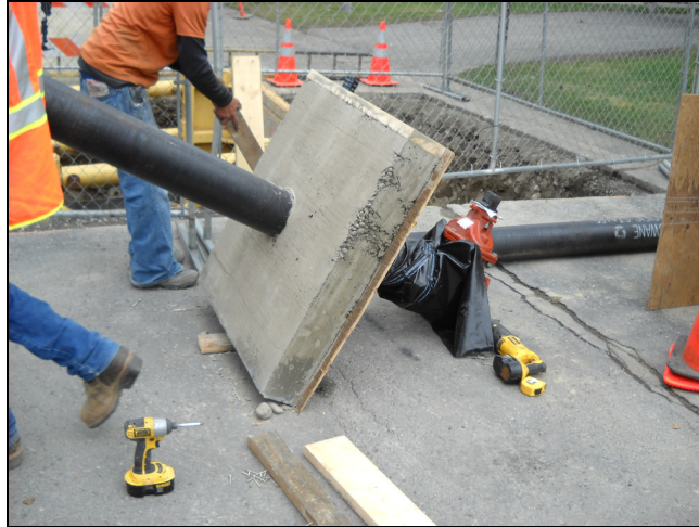
Figure 3. Thrust blocks are precast in some cases to minimize water shut-down times.
