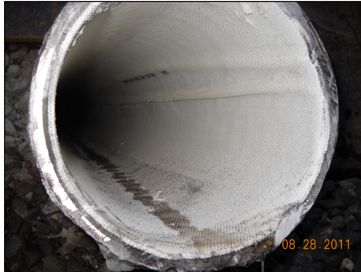
Figure 2. CIPP lined cast iron water main
