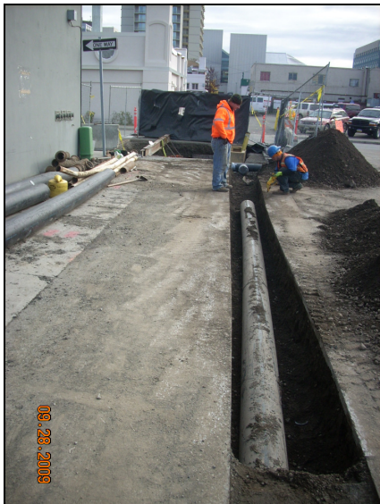
Figure 5. Buried temporary water piping in a business district.
