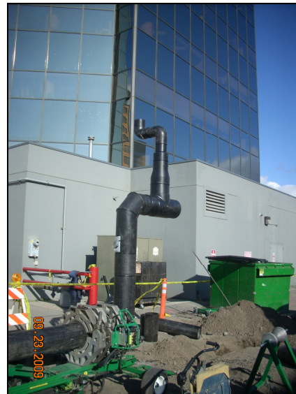
Figure 6. Elaborate pipe for a fire-flow sized temporary water system.
