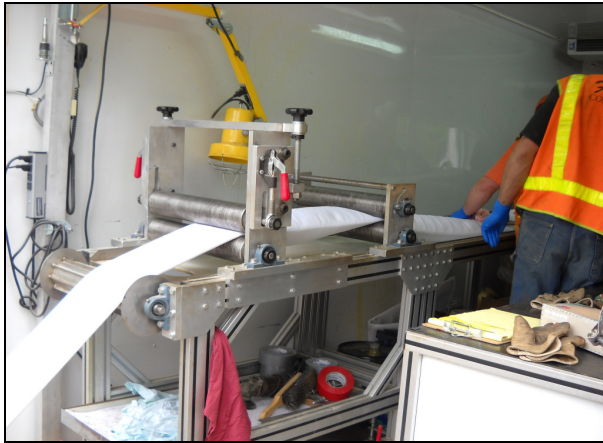
Figure 8. Wet-out and sizing equipment. Courtesy of Sanexen Aqua Pipe.
