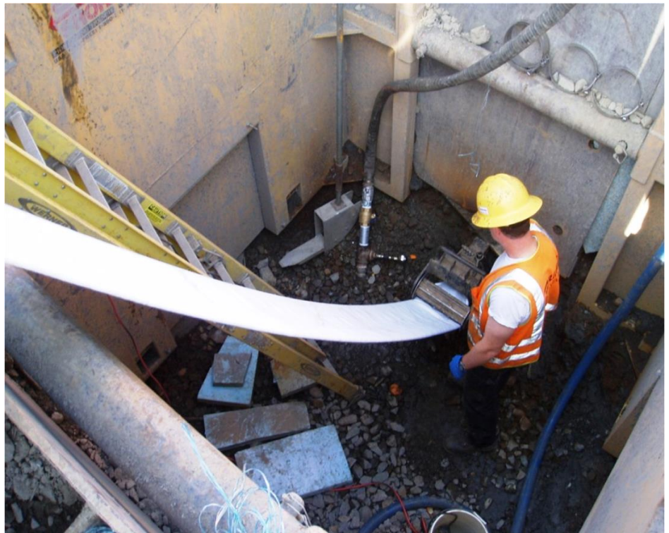
Aqua-Pipe is a structural liner that is designed and manufactured with mechanical properties exceeding all specifications and meeting drinking water requirements.
