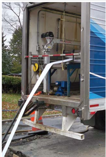
Installation of the structural cured-in-place liner.
