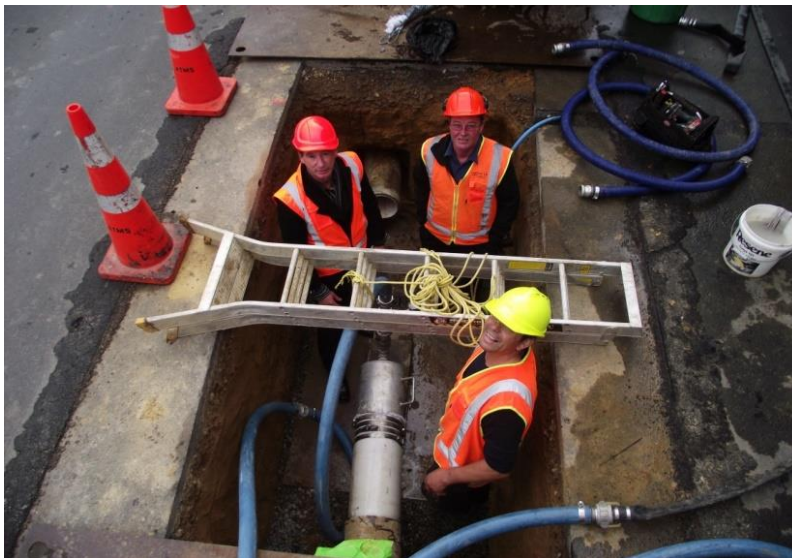
Relining Pit: ‘Pig Catcher’ in action, catching the forming swabs as they are propelled though the line during the forming and curing process
