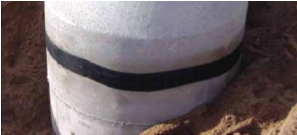
Aquawrap installed around a MH joint
